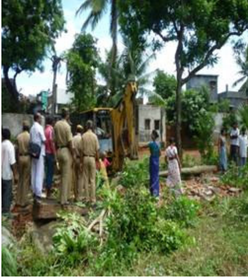
Demolishing dry latrine in Kurnool
